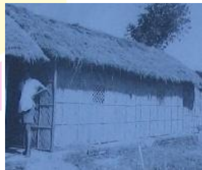
Bamboo house with thatch roof
