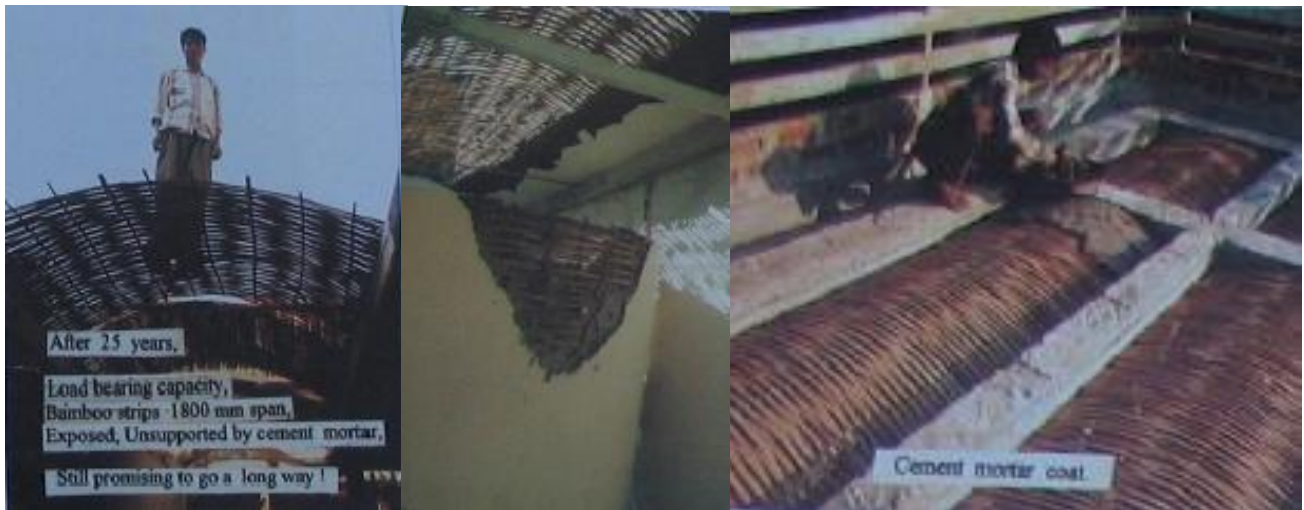
An experimental house with bamboo strips constructed during 1973
