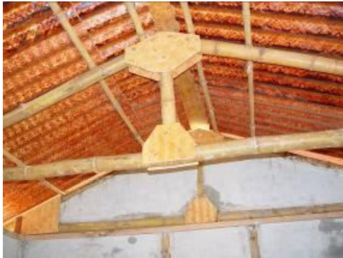
Fig. 2 Bamboo Trusses in a House
